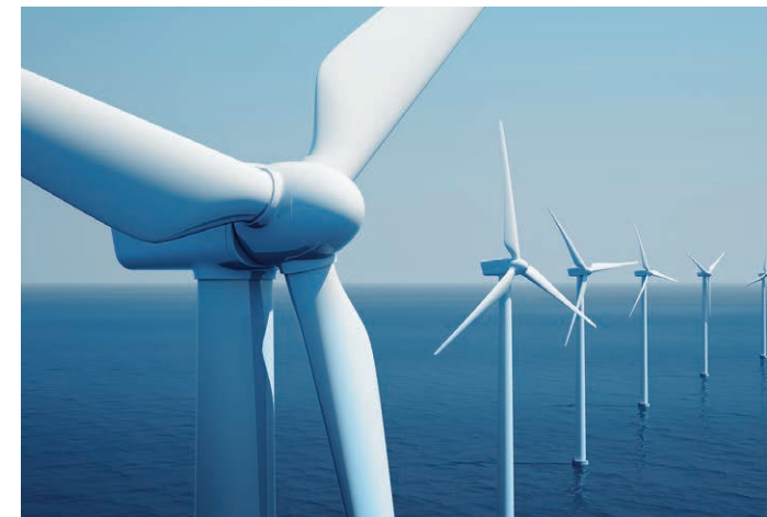
風力発電 Wind power generation
